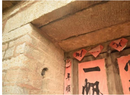
Fig. 6 Taian-Yin Shanzhuang: The lintel of the door is made of three different widths of stone. Chisel marks with straight or diagonal lines carved above the stone.
