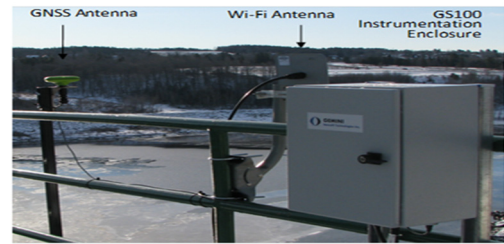
Fig. 2. GNSS Main devices for Fine Measurement on the bridge
