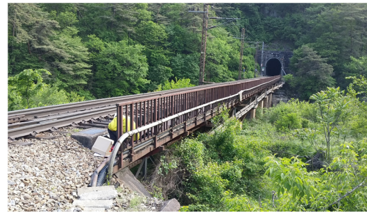
Fig. 6. USN/IoT Sensor Measuring on the railway
