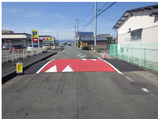
Figure 1. Example of a hump implemented in Saga-city [3]
