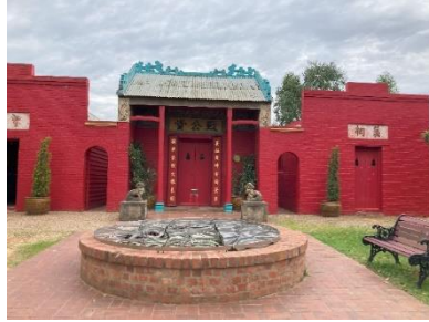
Figure 3. Bendigo Joss House Temple (exterior). Photograph by Author.
