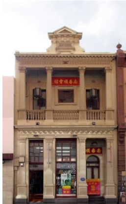
Figure 1. Num Pon Soon Building, Little Bourke Street, Melbourne. Wikimedia Commons
