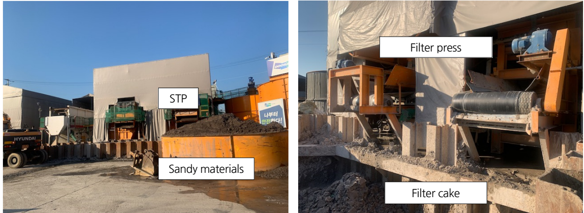
Fig. 6. Collection of material samples from slurry shield TBM project
