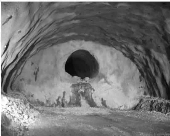
Photo 1. Photograph of cutting face of actual tunnel.
