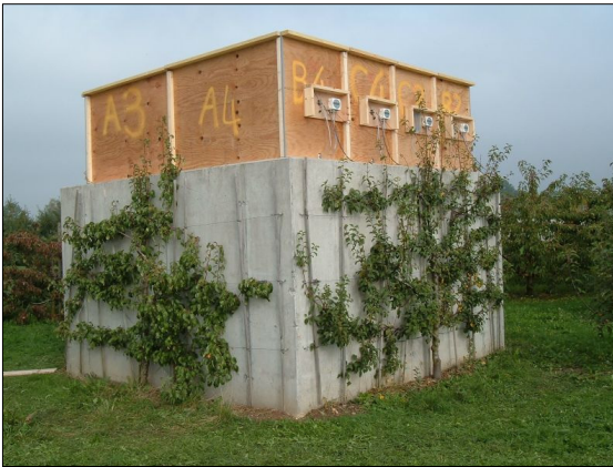
Fig. 5. Measurement enclosure on top of shaft
