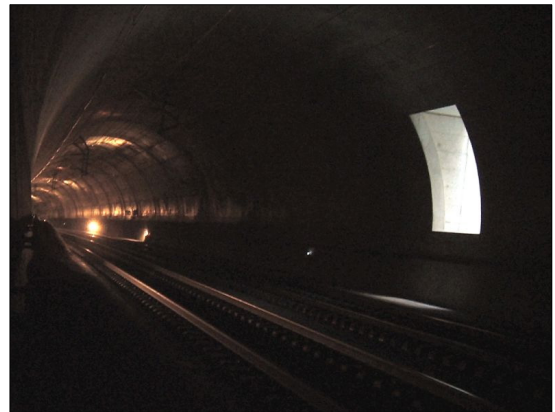
Fig. 2. Airshaft in Emmequerung tunnel
