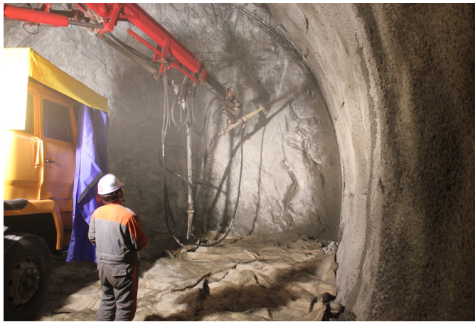
Fig. 7. Shoot the shotcrete
