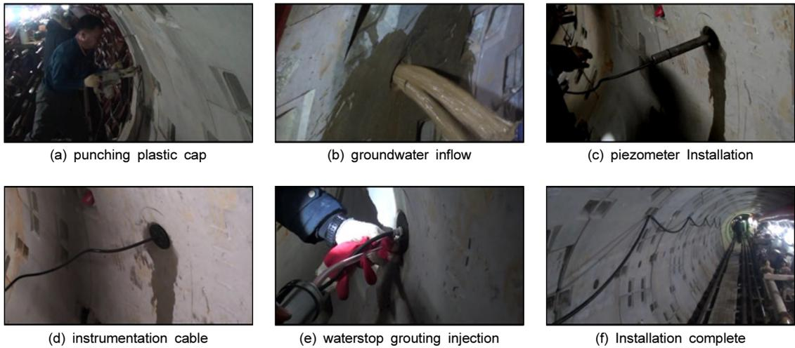
Fig. 12. Installation process of piezometer
