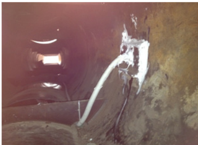
(c) Installation of sensor ③
