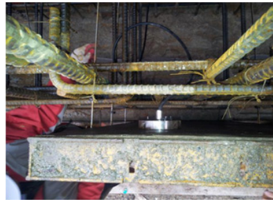
(b) Sensor④ on formwork
