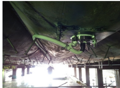
(b) Installation of sensor ②
