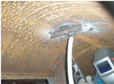
(a) Installation of sensor ①
