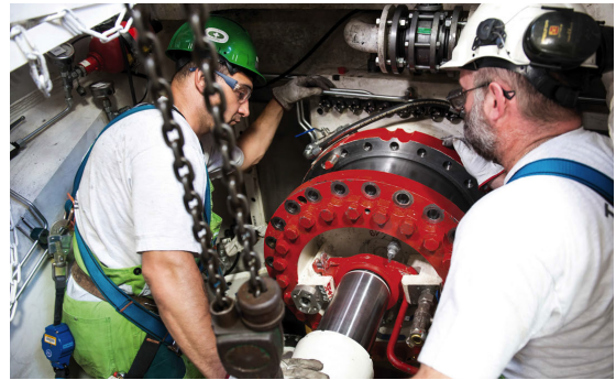
Fig. 8. Workers Changing Discs (Herrenknecht)
