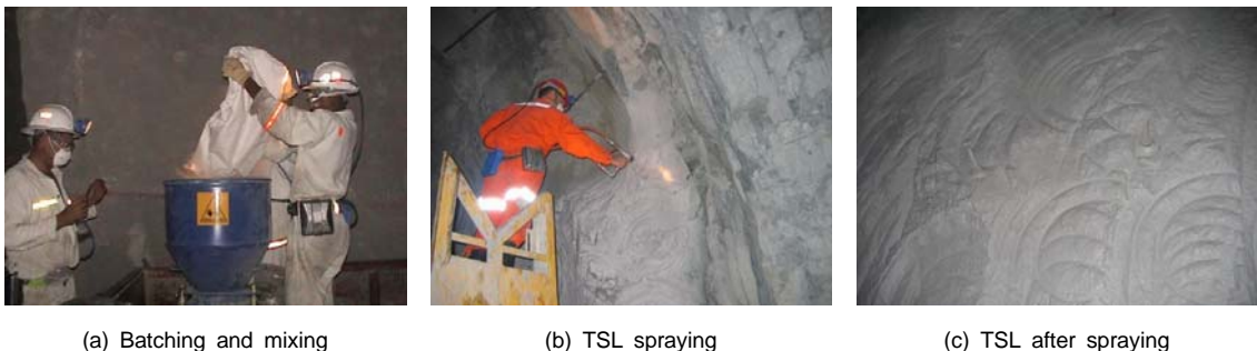
Fig. 1. Construction procedure of TSL (Saydam, 2008)
