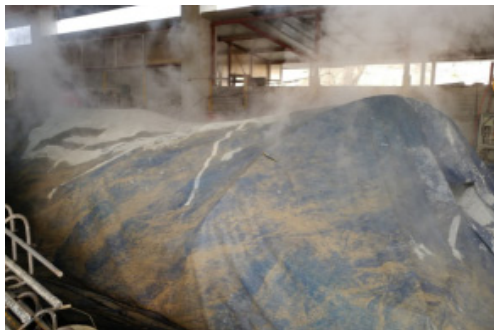
(e) Steam curing
