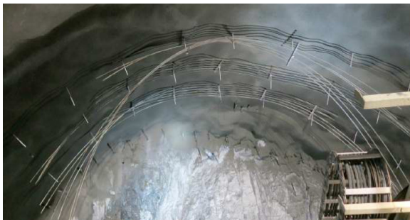
(a) Installation of RRS
