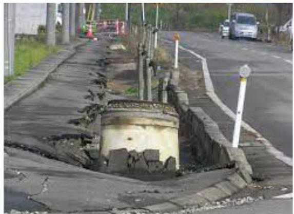
(b) Uplifted manhole and settled backfill
