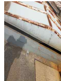
Figure 4: Rubber packing of aeration tank
