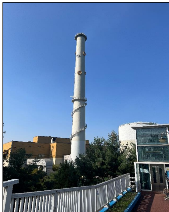
Figure 1: Gangnam Resource Recovery Facility
