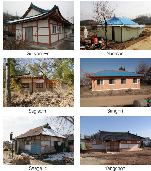
[Fig. 2] Picture of Secondary Station in Dangjin
