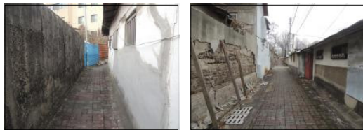
[Fig. 5] Side Street in Employee Residence Village
