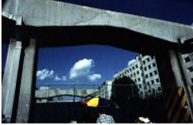
A section of the Samil elevated expressway under deconstruction, 2003 (© Ryu Jeh-hong)
