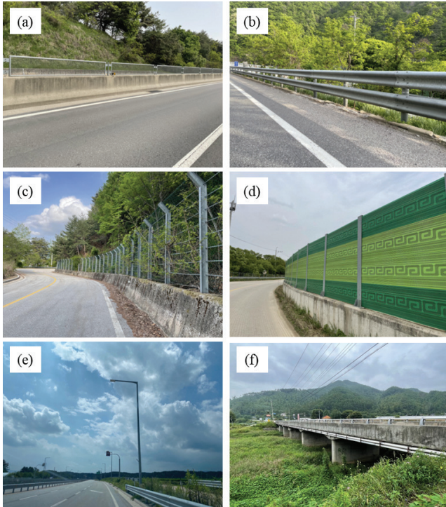
Fig. 2. Typical form of (a) bottom blocked median barrier, (b) bottom blocked guard rail, (c) rock fall fence (d) noise fence, (e) light and (f) bridge.
